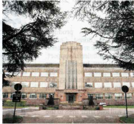
The site is an important example of Art Deco design.
